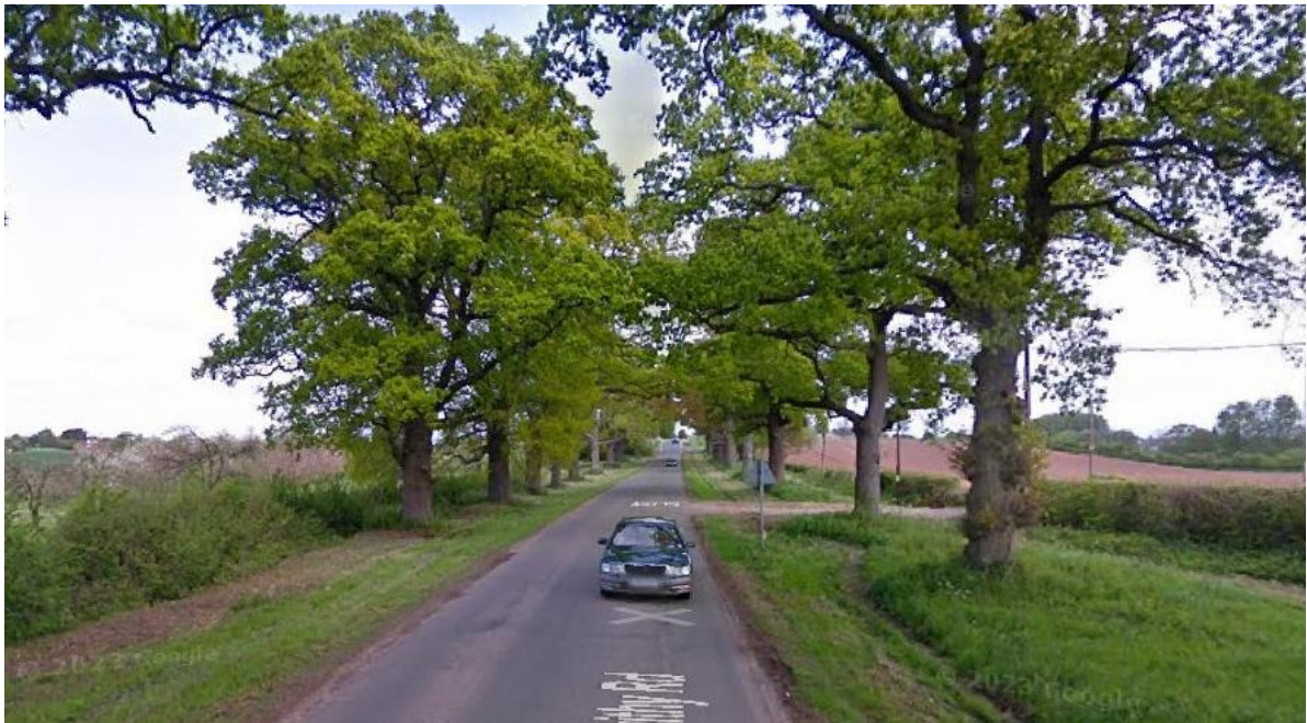
Figure 12: Existing Oak Avenue, approaching Green Crize.
